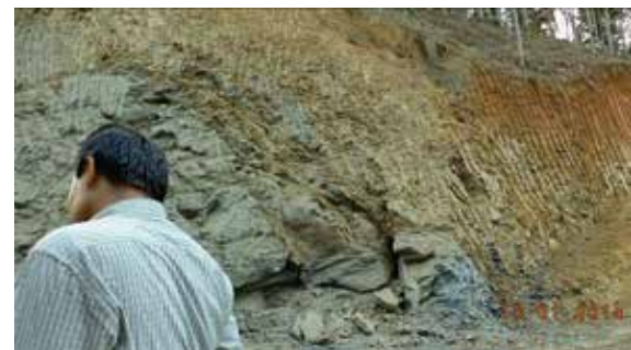
Figure 8 High angle shears traversing the rock mass in the cut slope
