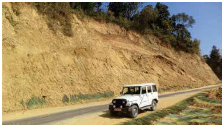
Fig. 15 Inclined rock soil interface – a site of probable translation failure during lubrication
