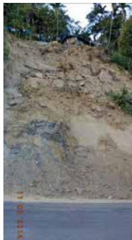
Figure 13 Prominent rock slide showing released boulder at vulnerable slope, Variengte
